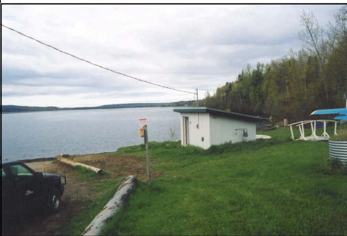
Plate 1. A view of the north end of Tabor Lake with the Tabor Lake Estates pump house in the center of the photo.
