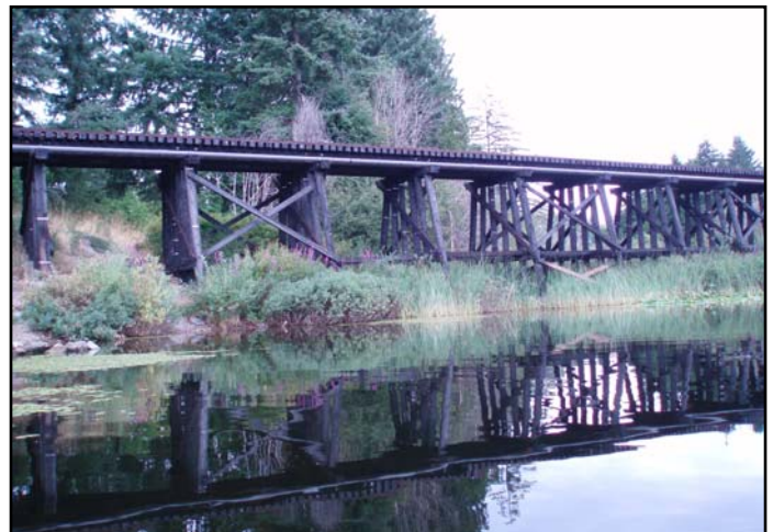
Photo 1: E & N railway trestle at north-end of Green Lake (MoE, 2008)
