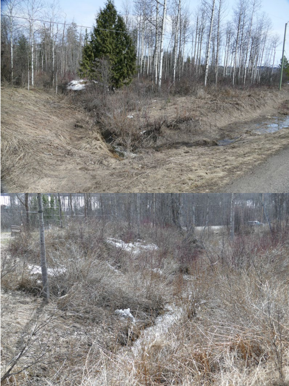
Figure B-5. Creek crossing Fisher Road near the octagon house looking southwest (above) and looking northeast (below).
