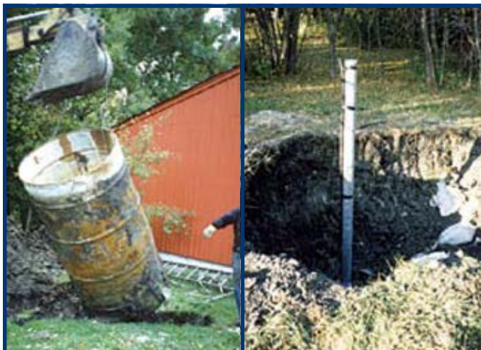
Figure 4. Well pit cribbing being removed by a backhoe
