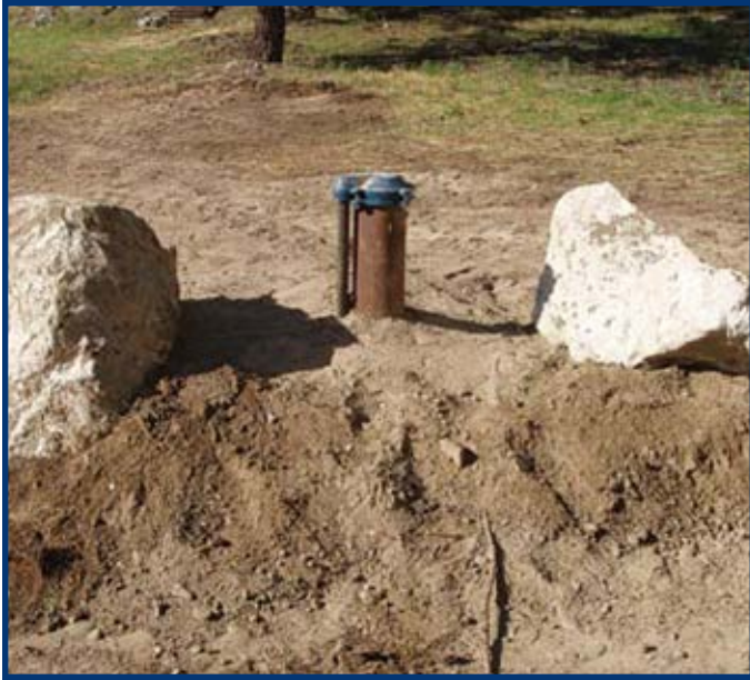
Figure 8. Grading around well head to protect well
