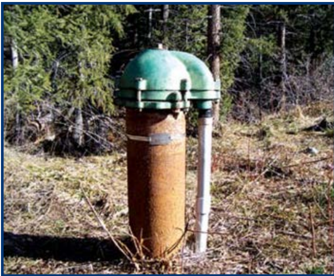
Figure 9. Secure well cap
