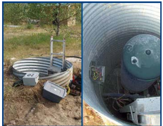
Figure 2. Well pit with metal cribbing
