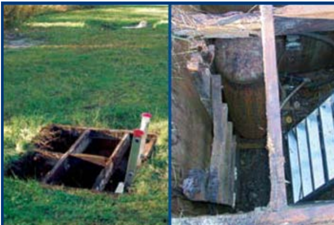
Figure 1. Well pit with wooden cribbing
