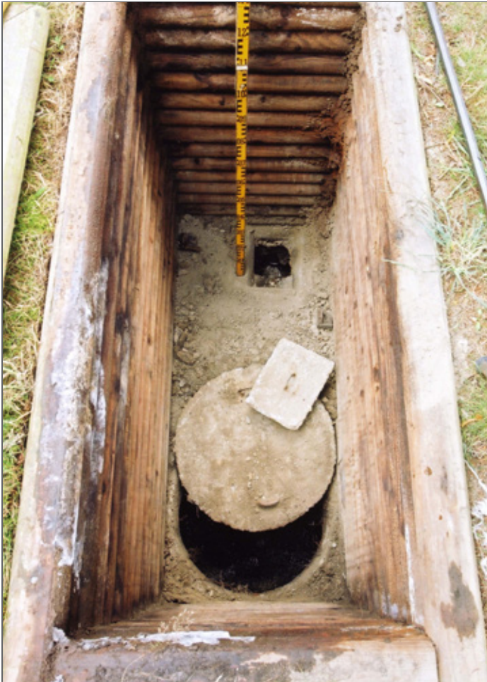
FIGURE 8 Deep septic tank in confined place (worksafeBC rules apply)
