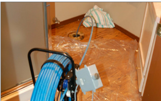
FIGURE 5 Using a pipe camera to find a septic tank
