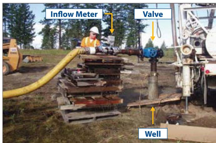
**FIGURE 3** In-line flow meter on discharge line
