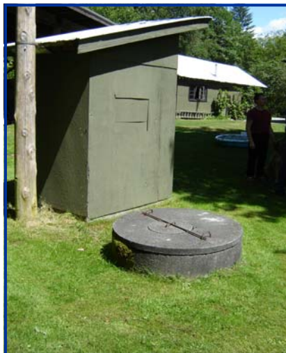
Figure 1: A typical dug well
