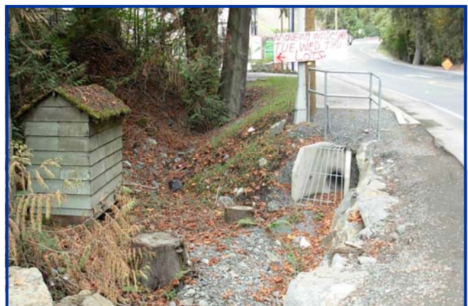
Figure 9: Dug well (in well house) near culvert & busy road
