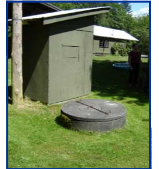
Figure 1: A typical dug well
