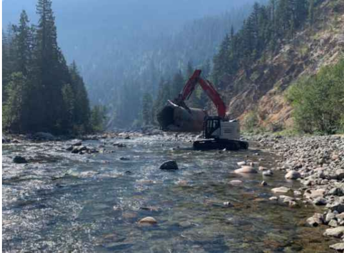
Culvert removal at TR-57
