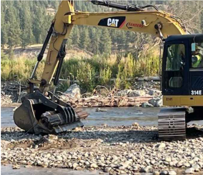
Misc. metal removal at NR-104
