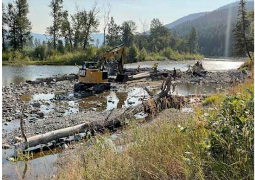
Concrete removal at NR-104
