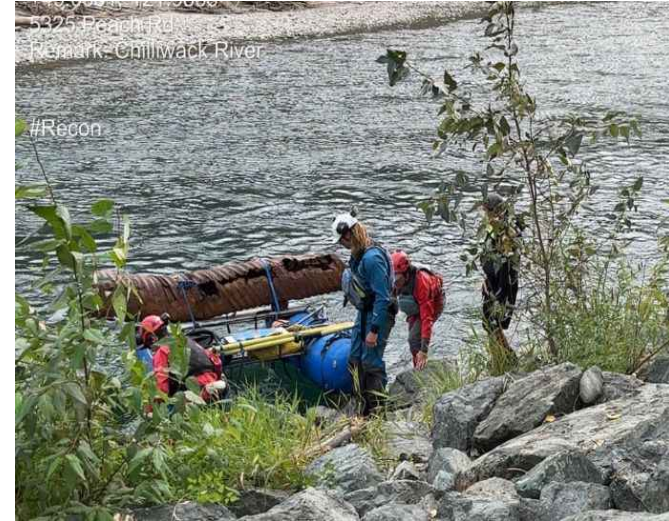
CH 60 removing culver using rafts
