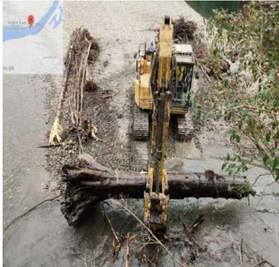
CH9 woody debris removal
