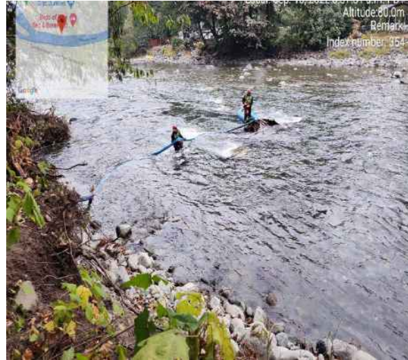
CH63 Culvert/ bridge pier towing
