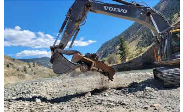
Excavator removing submerged vehicle at NR-72
