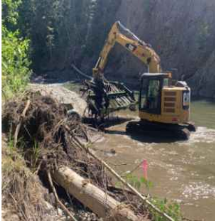
Removing farm equipment at CW-65
