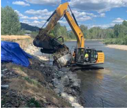
Removing vehicle out of Coldwater River.
