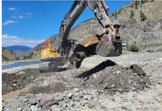
Excavator removing submerged vehicle at NR-72
