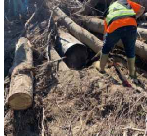
Removing metal at CW-74
