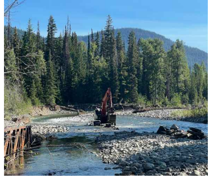
Concrete removal at Manning Park
