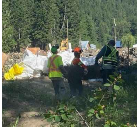
Linear debris work along Coldwater River
