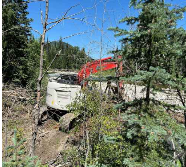
Manning Park bridge work
