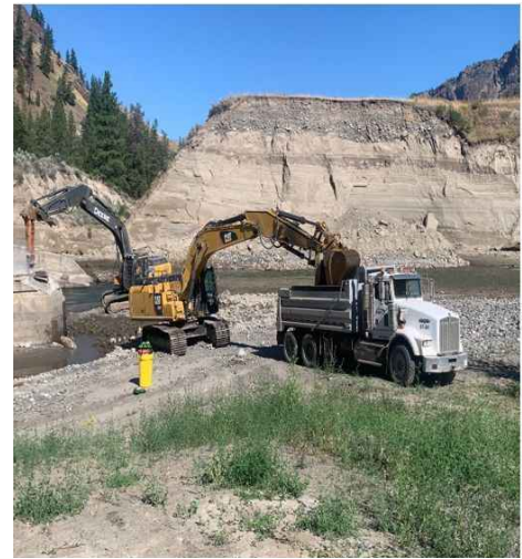
Breaking and loading out concrete at NR-80
