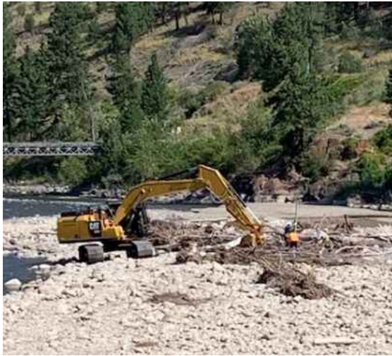
Debris removal at Nicola River
