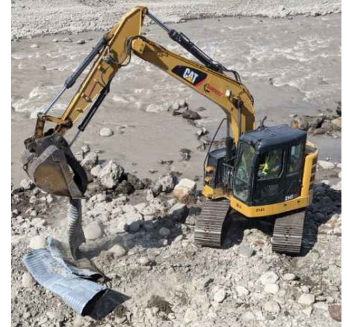
Removing culvert
