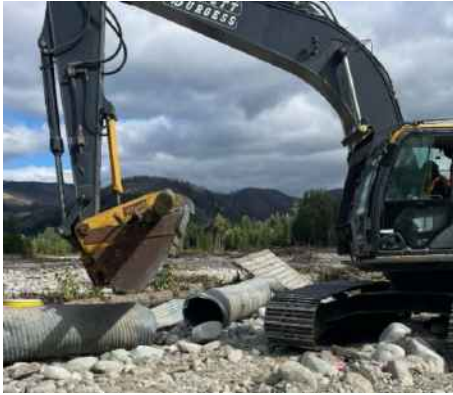
Culvert removal
