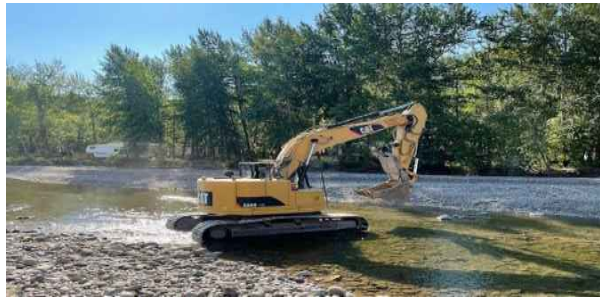
Misc. debris removal
