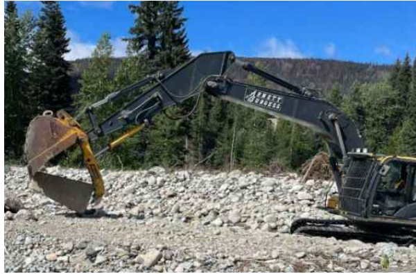
Concrete removal along Coldwater River
