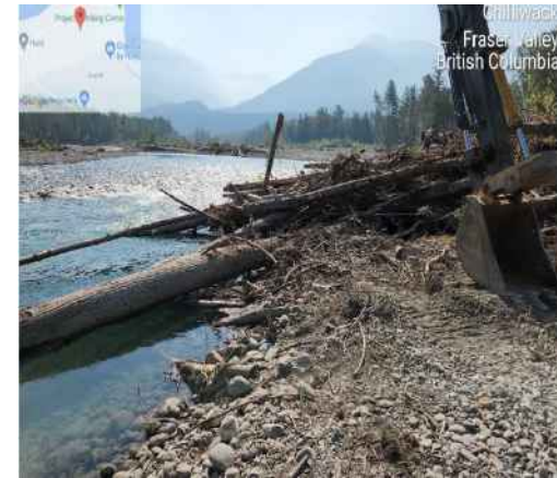
Continuing work CH10
