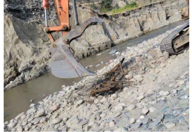
NR-73 debris removal of metal
