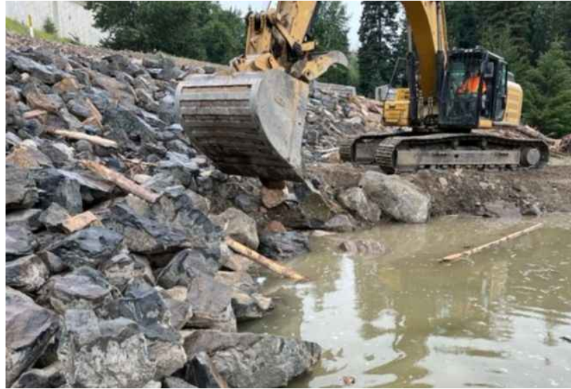
CW-66 concrete abutment removal and clean up
