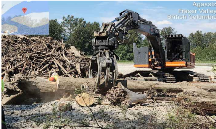
Woody debris removal FR 10
