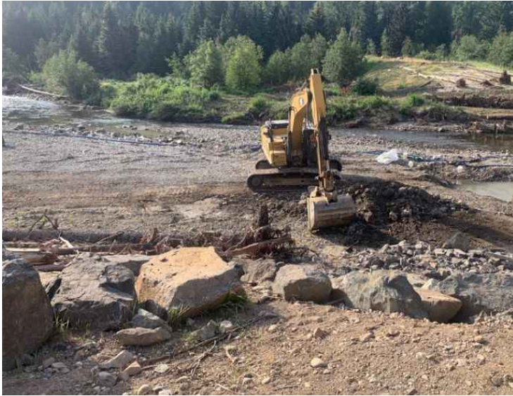
CW-66 concrete abutment removal and clean up
