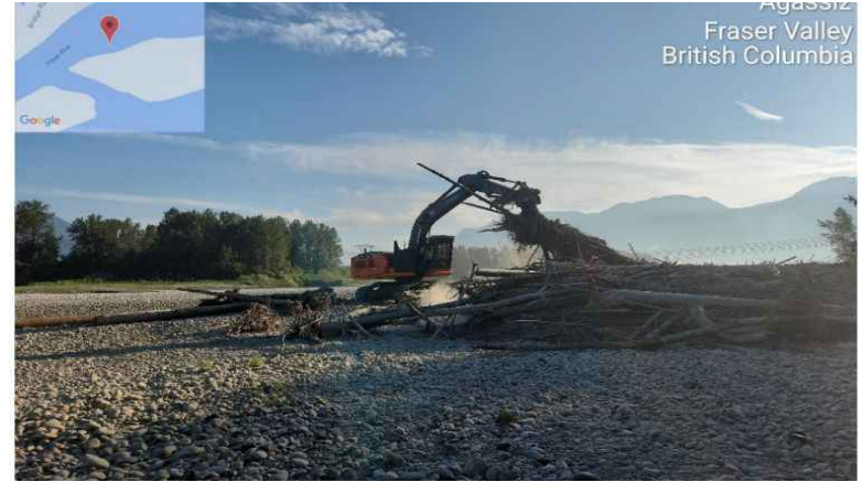
Woody debris removal FR 10
