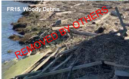
REMOVED BY OTHERS (REPAIRED)
