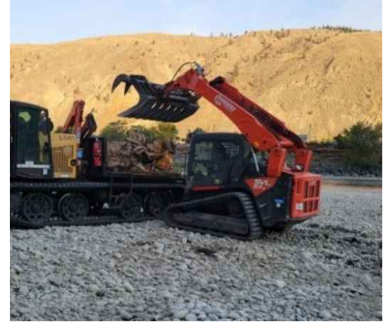
Debris being loaded for removal
