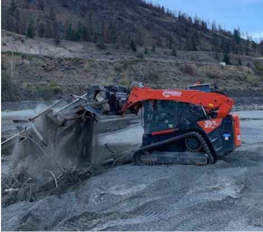
Debris removal along Thompson River
