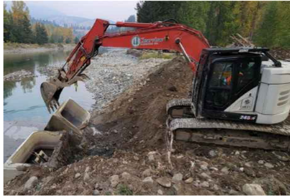
Concrete intake removal at TR-100
