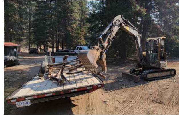
Loading of metal debris
