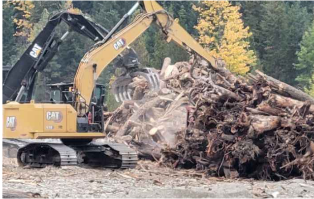
Woody debris removal at TR-84
