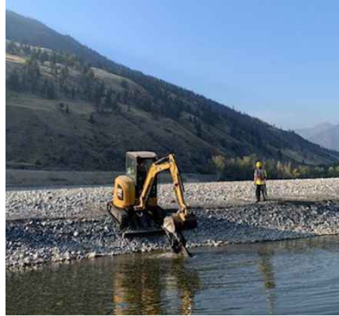
Removing debris from Thompson River
