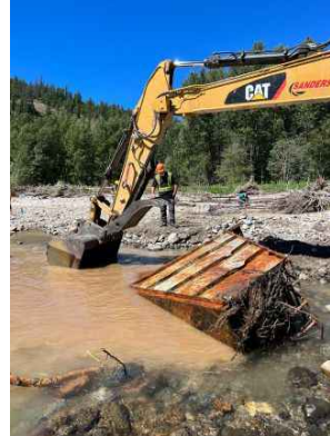
Metal objects removal at CW-39
