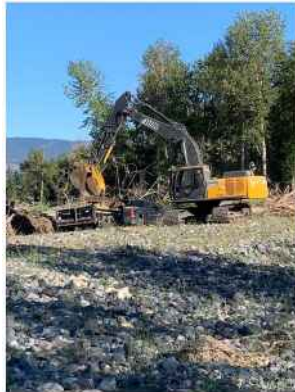
Debris removal at CW-51
