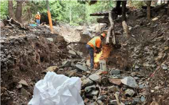
Making access to Rockwell Drive
