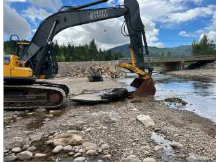
Camper removal at CW-54
