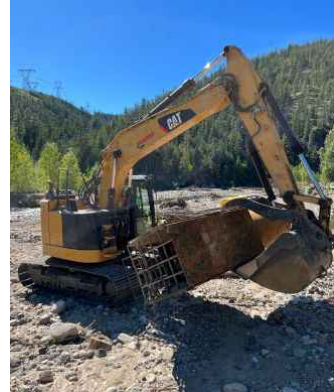
Metal objects removal at CW-39
