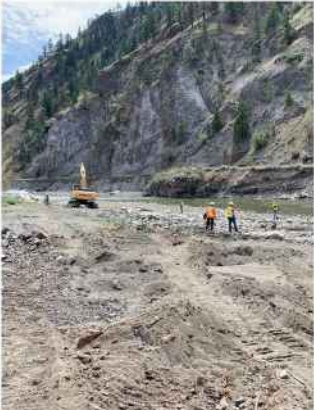
Debris removal at NR-71
