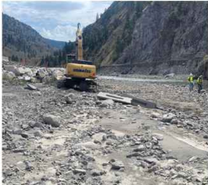
Debris removal at NR-71
