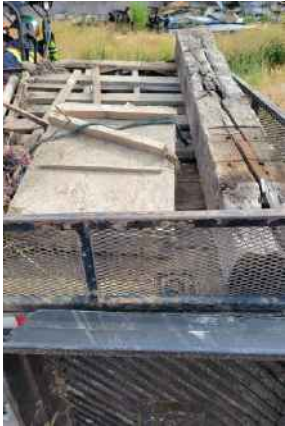
Debris removal at NR-83
