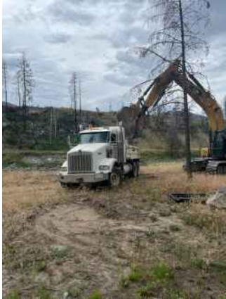
Hauling debris at NR-83
