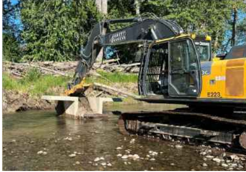
Concrete structure removal at CW-51
