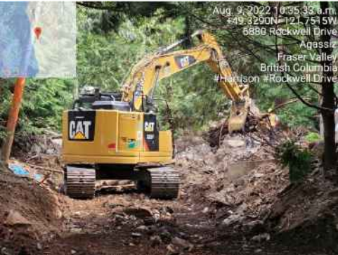
Removing debris at Rockwell Drive
