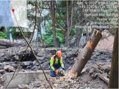
Removing debris at Rockwell Drive
