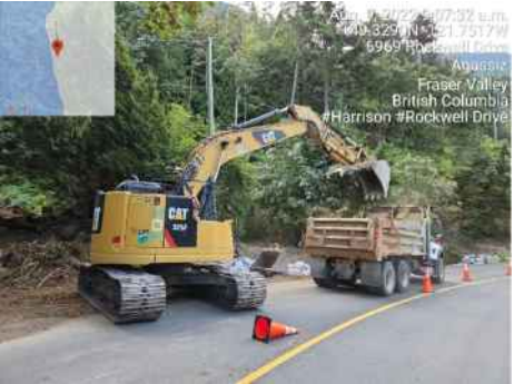
Removing debris at Rockwell Drive
