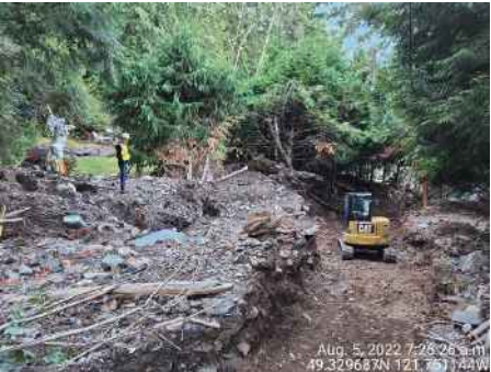
Making access to Rockwell Drive
