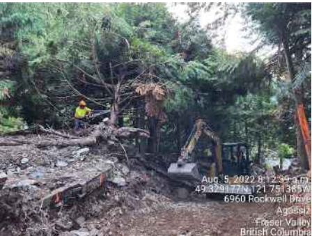
Making access to Rockwell Drive
