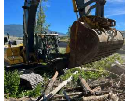
Concrete structure removal at CW-51
