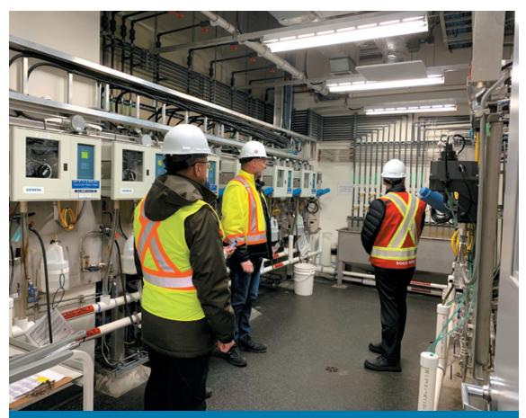
A certified EOCP Operator providing a tour of the analyzer/sampling room of the Seymour-Capilano Water Filtration Plant in North Vancouver. Water from different stages of the water treatment process are plumbed to this room for easy dedicated sample collection and to online analyzers for chlorine residual, pH, conductivity, and UV transmittance. Photo credit: Environmental Operators Certification Program.
