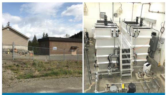
The MacArthur-Reedman water treatment plant and reservoir (Left), owned and operated by the Columbia-Shuswap Regional District. Inside the water treatment plant (Right). A small water system successfully achieving the BC surface water treatment objectives through two direct filtration pre-packaged plants, UV, and chlorination. Photo credit: Columbia-Shuswap Regional District.
