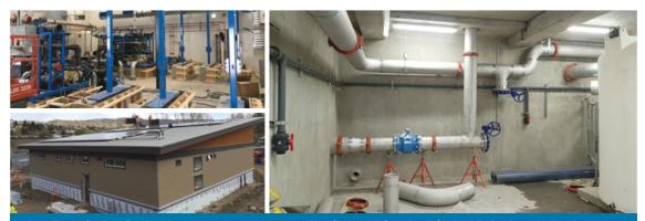
The Village of Ashcroft is building a new water treatment plant (bottom left and right) scheduled to be completed in late summer 2019. The new facility will be equipped with membrane filtration (top left) and a new chlorination system providing primarily disinfection. With the upgrades, the Village will provide potable water that achieves the BC surface water treatment objectives. Photo credit: Maple Reinders Constructors Ltd.
