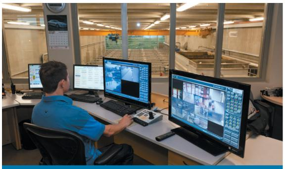
View from the Kamloops Centre for Water Quality Operators Control Room where they have the Supervisory Control and Data Acquisition (SCADA) system and security monitors. Operators can conduct all process operations of the facility from this room. Photo credit: Olsen Imaging.
