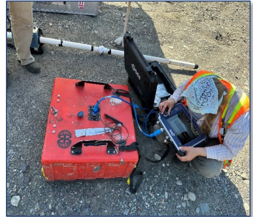
Photo 3: Electromagnetic (EM) mapping reduces unnecessary disturbance to the dam.
