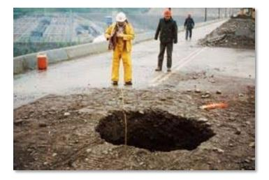
To investigate the condition of the dam core, a Becker drill was brought on site. After advancing the pipe with very little resistance to a depth of 32 m, the drillhole began to open up, resulting in a cavity approximately 2.5 m in diameter and 7 m in depth. A second smaller void associated with another survey benchmark was later discovered.
