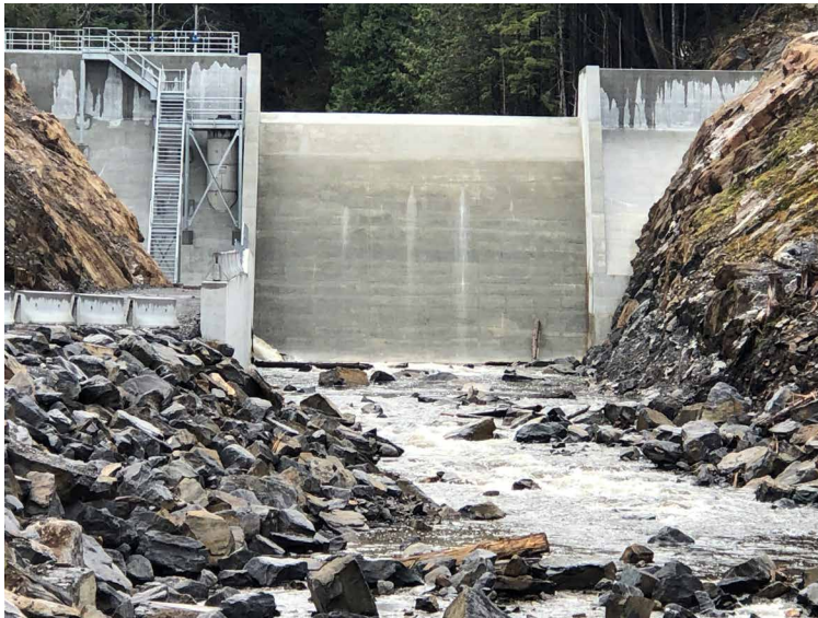
Photo 8 – New Woodworth Dam – looking upstream
