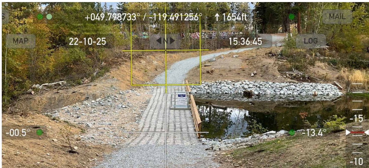
Photo 9 – Fraser Lake Dam with new spillway
