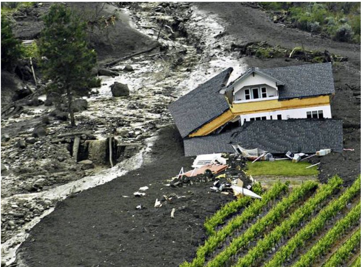
Photo 4 – Testalinden Dam failure consequences.
