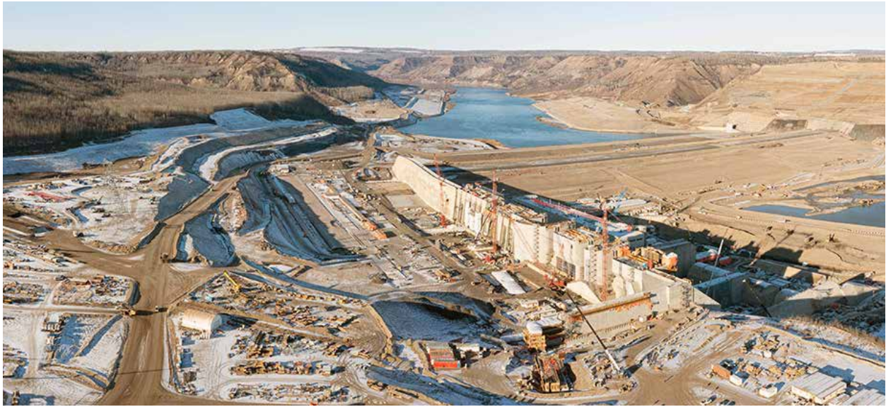
Photo 6 – Site C – An upstream view with the approach channel at left, and the powerhouse, generating station, and the earthfill dam at centre. (Photo credit: 2017 Site C Clean Energy Project)
