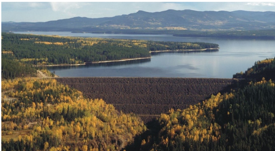
Photo 1 – Kenney Dam – Nechako Reservoir (credit Rio Tinto)
