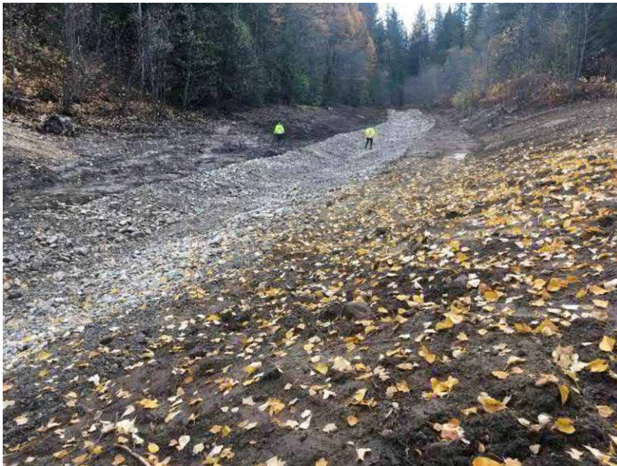
Photo 11 – Rehabilitation of stream channel following the removal of the East McDermid Creek Dam (credit: Masse Environmental Consultants Ltd)
