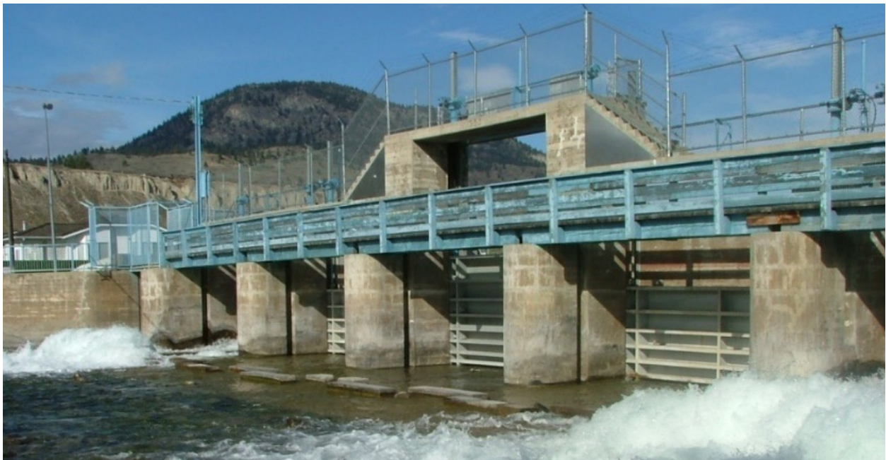
Photo 3 – Okanagan Lake Dam constructed for flood control purpose.
