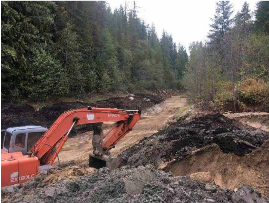
Photo 10 – East McDermid Creek Dam removal process (credit: Masse Environmental Consultants Ltd)
