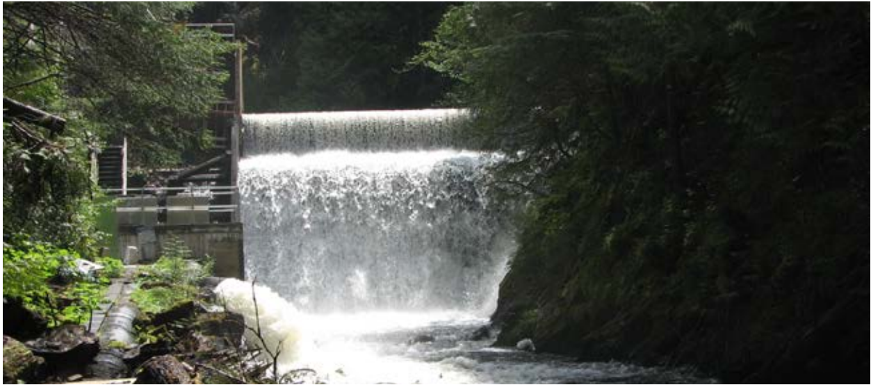
Photo 9 – Original Woodworth dam
