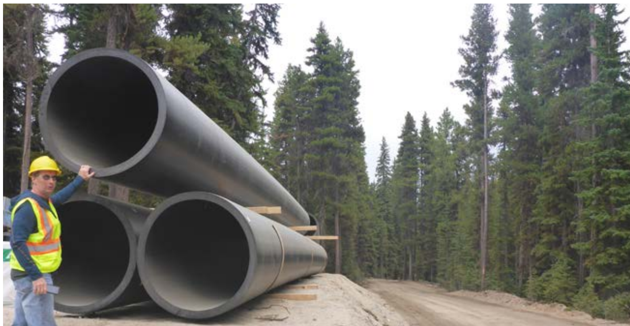
Photo 11 – New pipe to be installed
