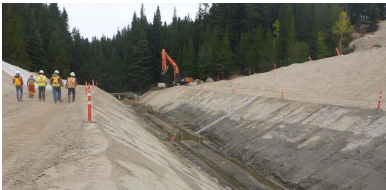
Photo 12 – Isintok Lake Dam with low level outlet pipe removed
