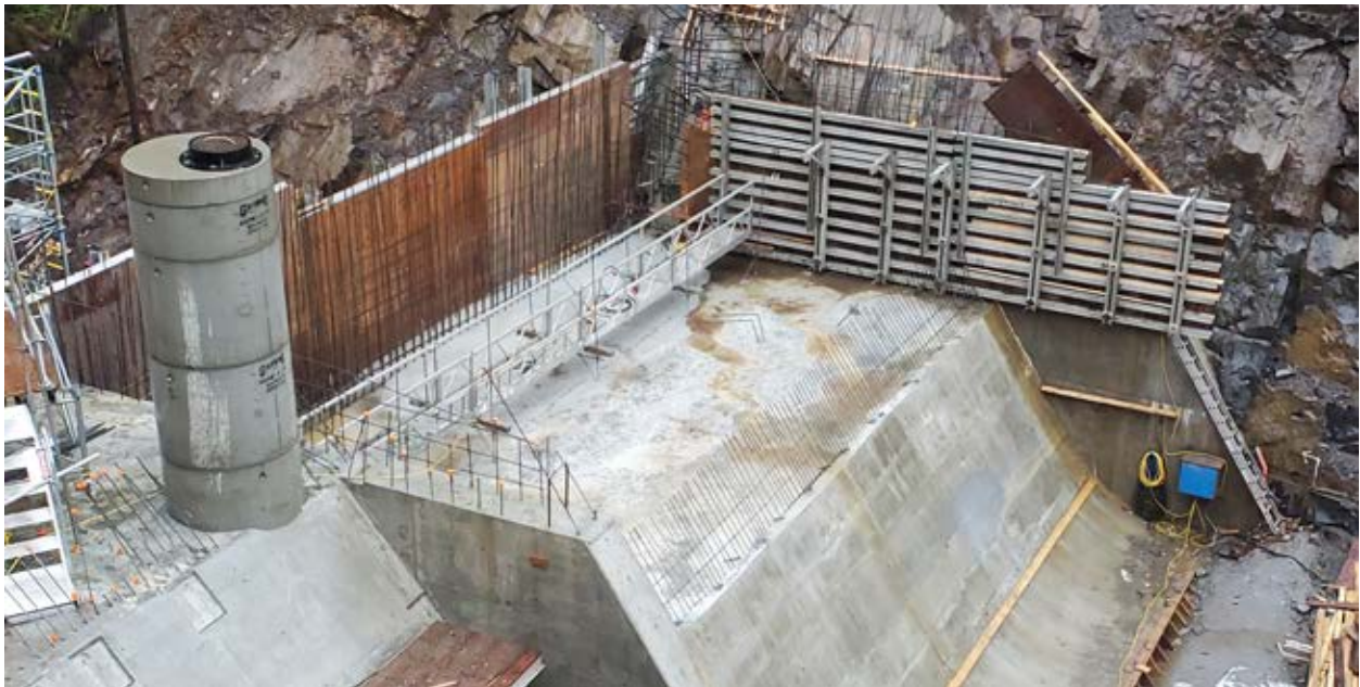
Photo 10 – Construction of new dam
