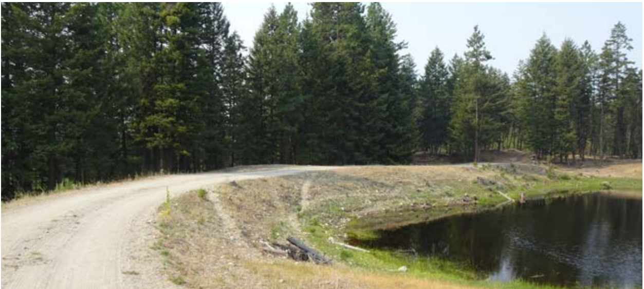
Photo 2 - Lower McCuddy dam
