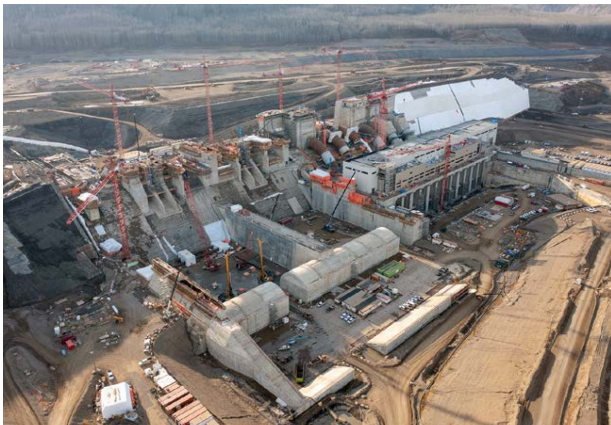
Photo 8 – Site C – Spillway, Powerhouse and RCC Buttress (Photo: BC Hydro)
