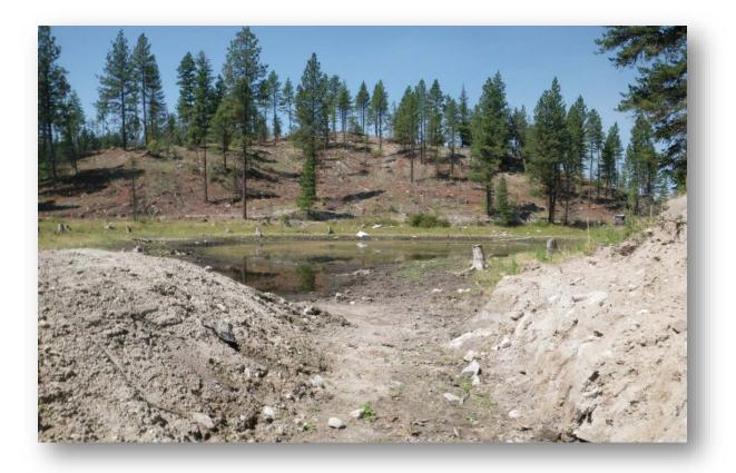
**Photo 3:** Decommissioning of small off-stream dam.
