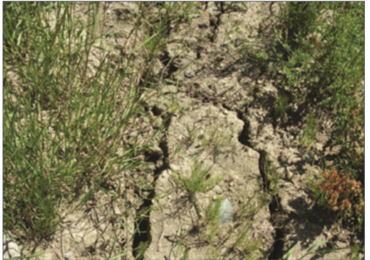
Transverse Cracks Indicate Dam Instability
