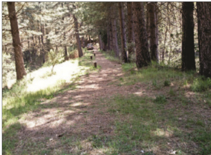
Trees Growing on the Crest and Faces of the Dam
