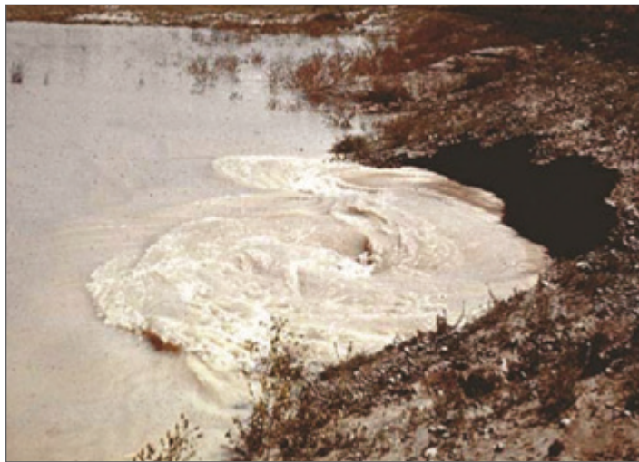
Whirlpools Indicate Advanced Piping Issue
