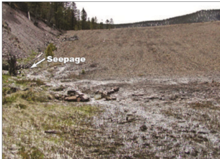
Abutment Seepage May Lead to a Dam Failure
