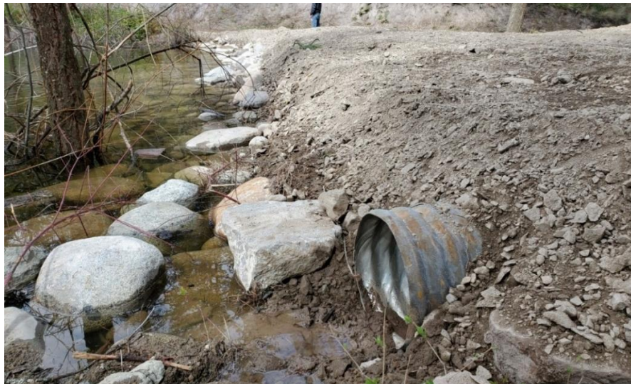
Photo 9: Unauthorized regulated dam with recently added culvert spillway of unnamed lake northwest of Okanagan Falls.
