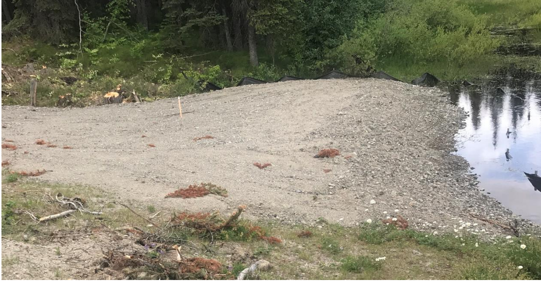
Photo 13: Repaired boil at Headwaters #1 Dam. Photo taken on July 24, 2020.
