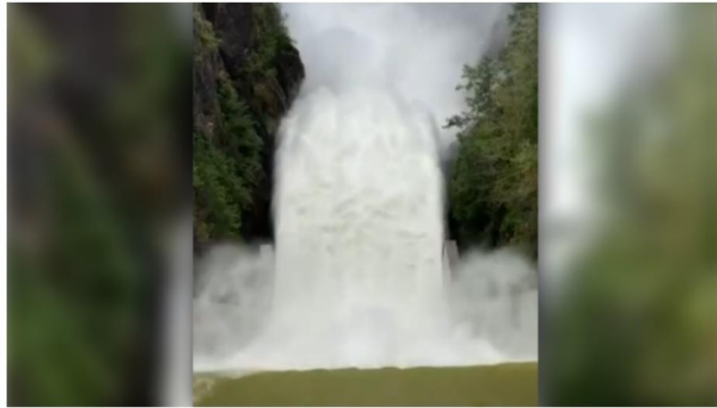
Photo 14: Uncontrolled release of water from the Cleveland Dam, October 1, 2020 (Credit: Twitter/Christine Tam)
