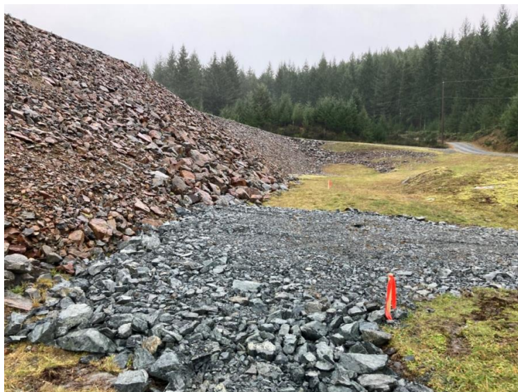
Photo 15: Filled depression at toe of Sooke Lake Dam where seepage collected
