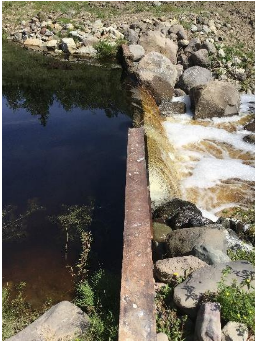
Photo 10: Rock reinforcement of the Willan Lake weir dam
