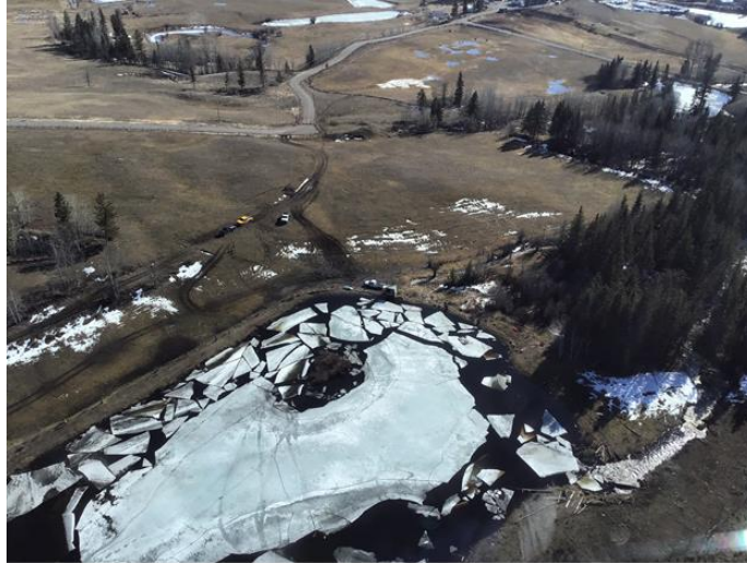
Photo 1: Overtopping and erosion of the Valley Pond (Upper) Dam embankment
