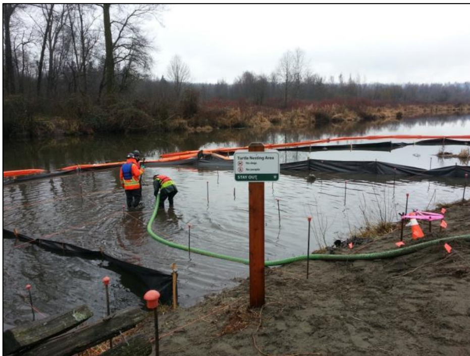
Photograph 16: Quantum crew beginning coal recovery after salvage was complete
