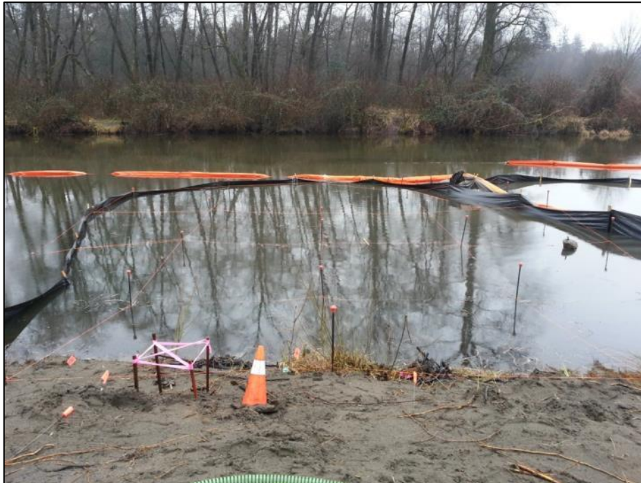
Photograph 17: South facing view of the recovery area and established grid for coal recovery adjacent to the turtle nesting beach
