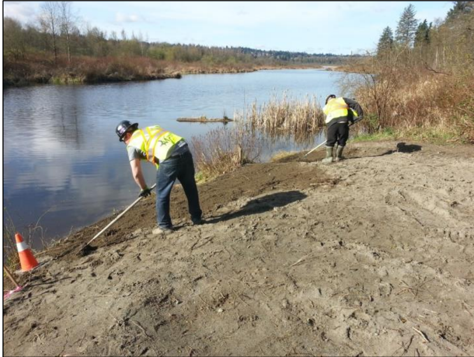
Photograph 23: Crew raking up the turtle nesting beach to reverse any compaction which might have occurred. The beach sand was raked to a depth of 100 mm to 200 mm, depending on the depth of the base material.
