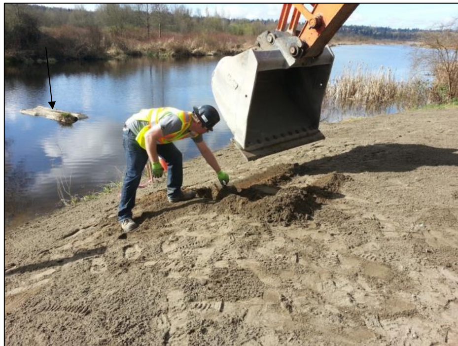
Photograph 24: Crew removing stump found in the turtle nesting beach
