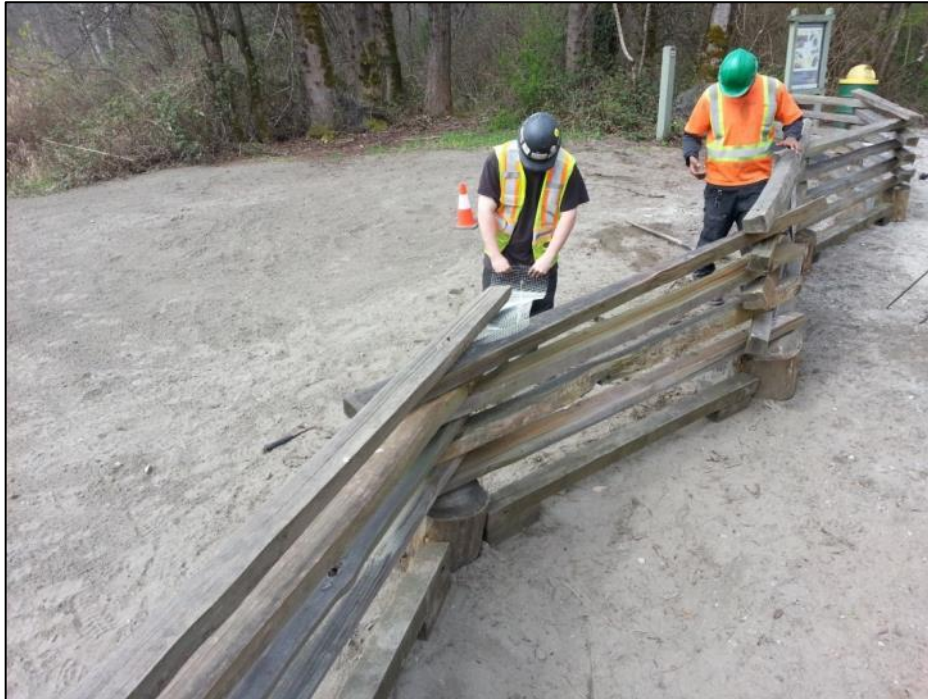
Photograph 29: Northwest facing view of the turtle nesting beach, crew installing the exclusion fence
