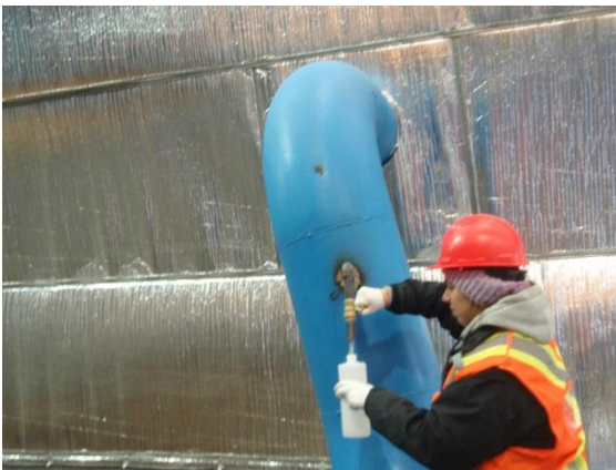
Photo 3. Effluent from discharge pipe (HAD-03)
