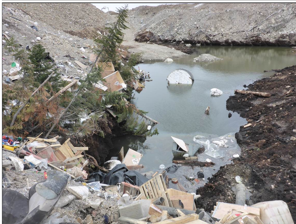
Figure 2. Since the last inspection on 14 June 2016, an area has been excavated to the rear of the site. Following freshet, this hole has filled with water and waste material was observed floating in it. An oily sheen was evident at the downwind end of the pool.
