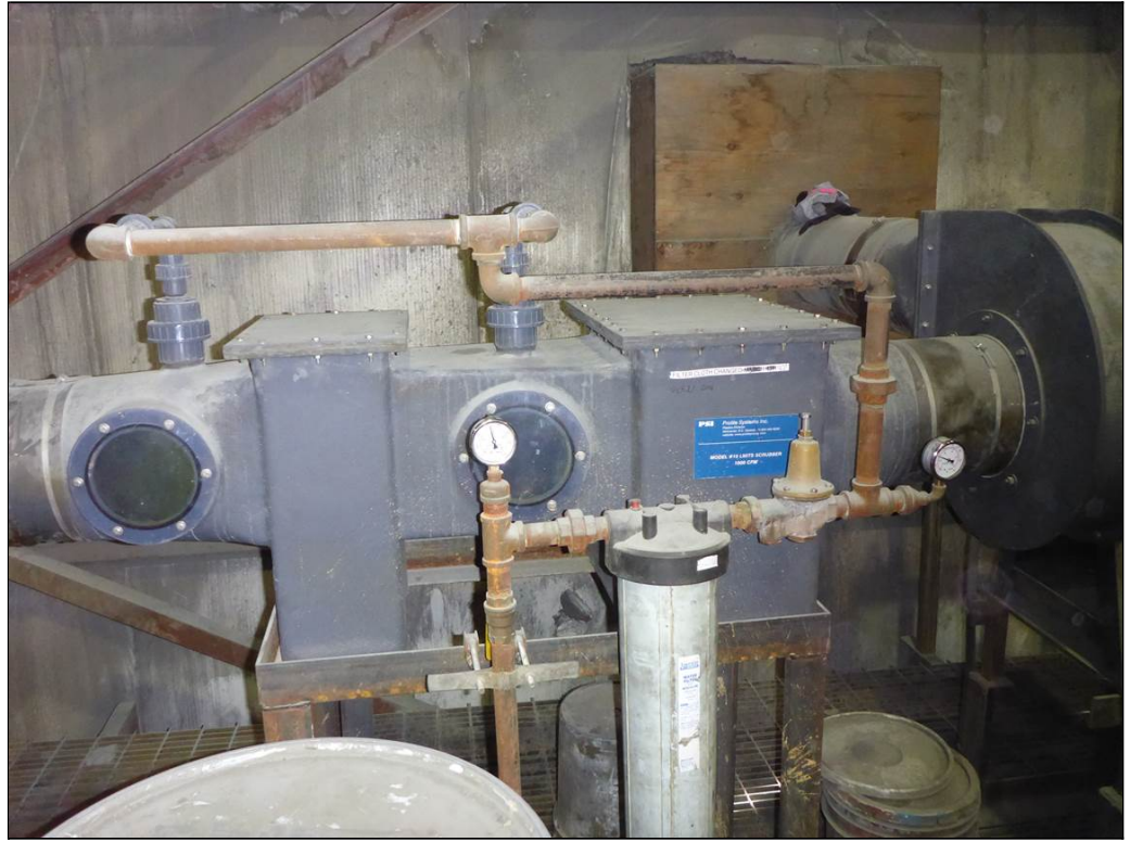
Figure 1. Wet scrubber treating emissions from the Reagent Mixing and Storage Tank Vents.
