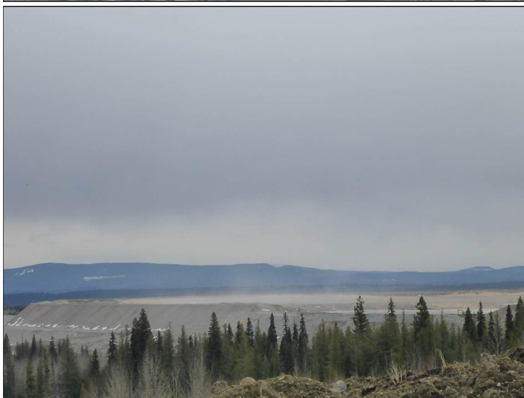
Figure 4. Wind blown fugitive dust generation on the TSF.
