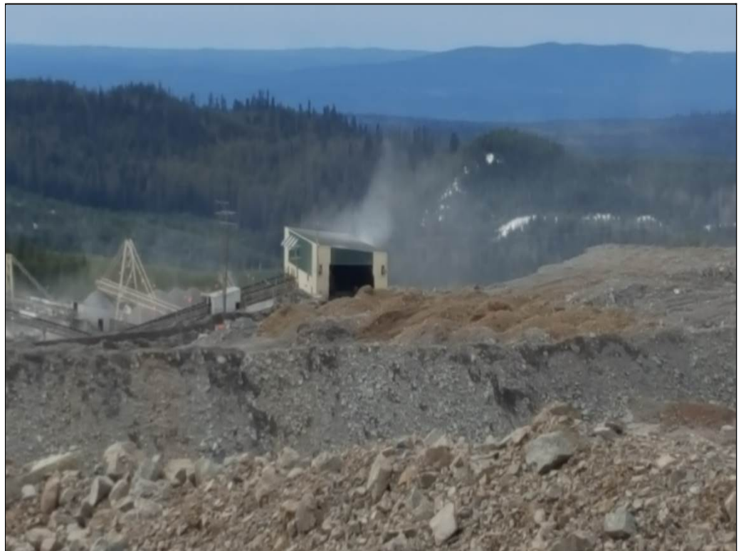
Figure 2. Fugitive dust emitting from the Crusher and Screening Plant discharge.
