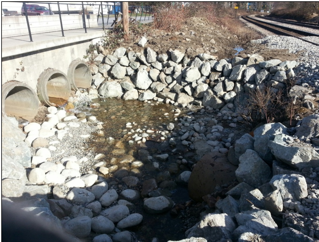
Photo 1. City of Burnaby storm sewer outfall upstream of the railway ROW
