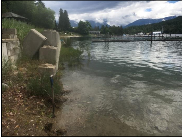
Photo 1. Section 1 - Upstream view.
