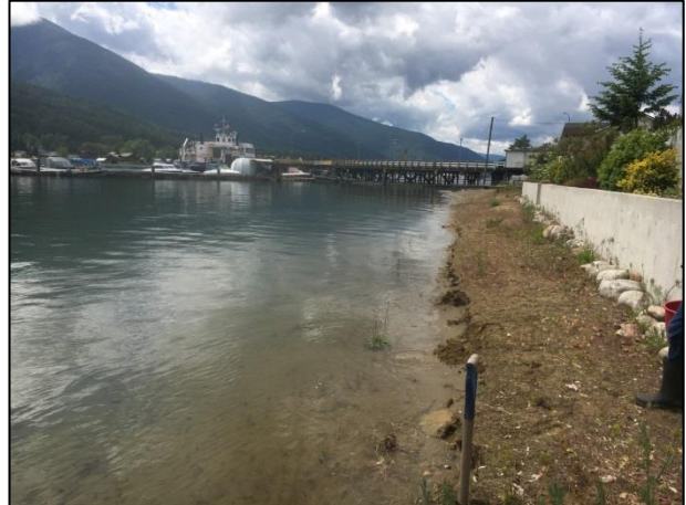
Photo 2. Section 1 - Downstream view
