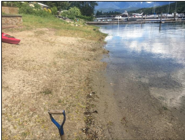
Photo 9. Section 6 – Upstream view.
