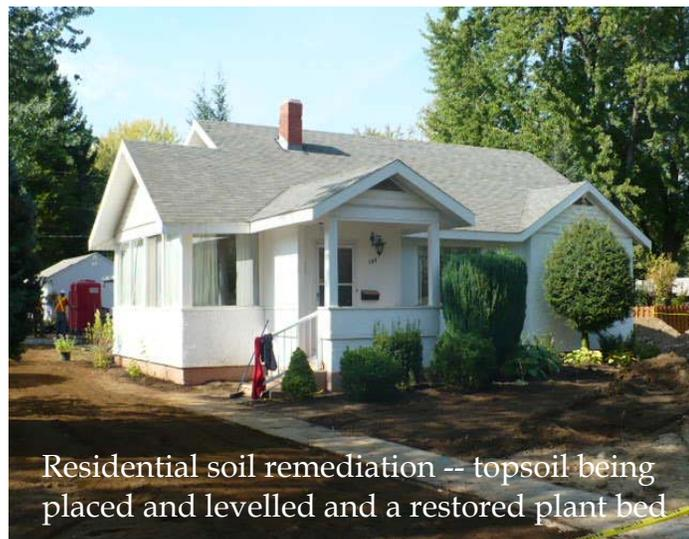
Residential soil remediation -- topsoil being placed and levelled and a restored plant bed
