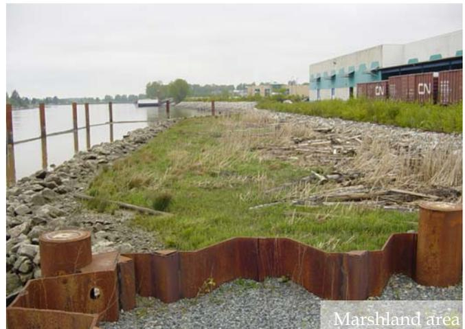
and control groundwater. Connecting the walls was an innovative “cap,” consisting of a protective sand and gravel layer, over which was a low permeability layer of clay-like material called Aquablok, and finally another
