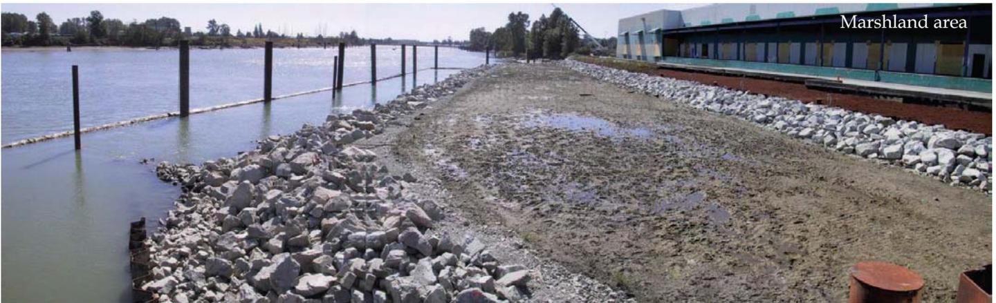
sand and gravel layer. The cap acted as the foundation for a constructed marshland area, and a shoreline extension was developed into a riparian habitat. Structural features included offshore densification piles for seismic resistance and both onshore and offshore berms to provide stability and erosion protection.
