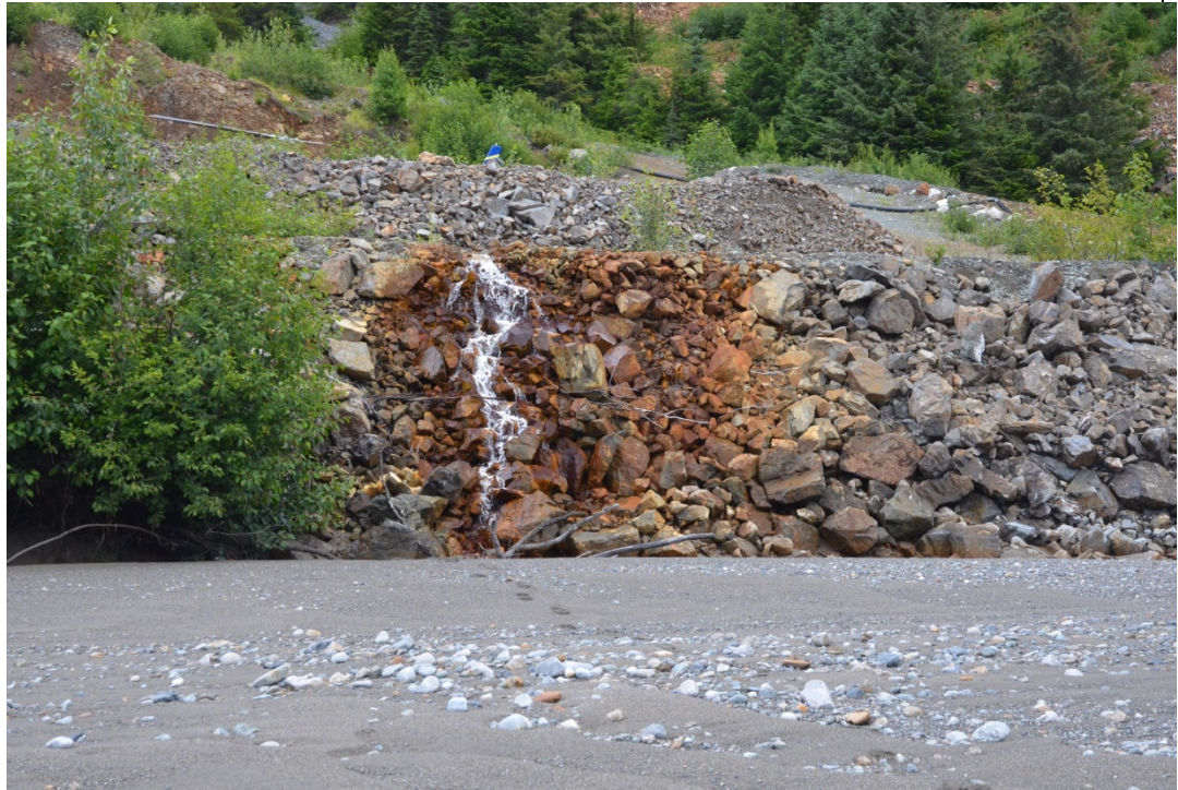
Photo 5 Effluent overflowing from the exfiltration pond.
