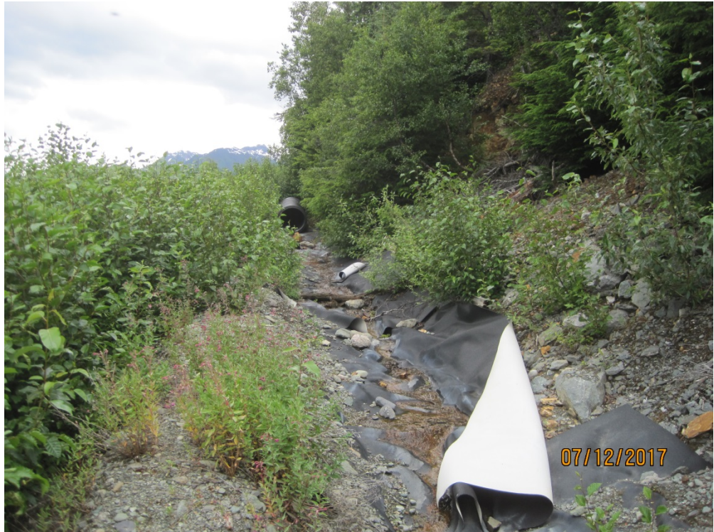
Photo 9 There is very little flow exiting the Portal Creek Diversion.
