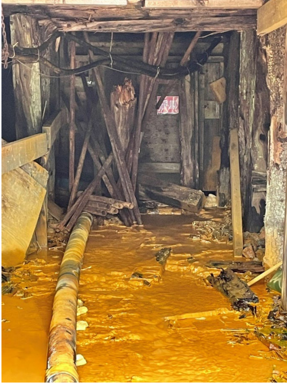
Figure 6: Entrance to the 5400 portal, showing the door at the back and fallen debris blocking access and indicating the need for additional structural fortifications.
