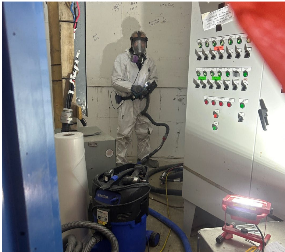
Figure 10: Mold abatement work conducted inside the water treatment plant.
