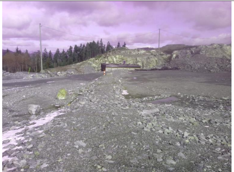
Leak and leachate detection works
