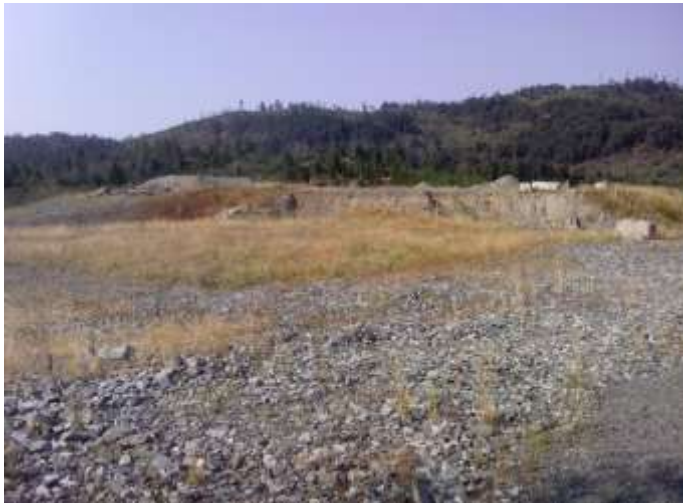
Contact water containment Pond
