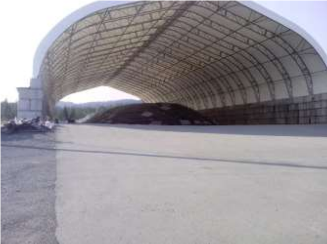
SMA - looking south
