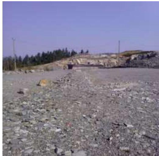
Leak and leachate detection works
