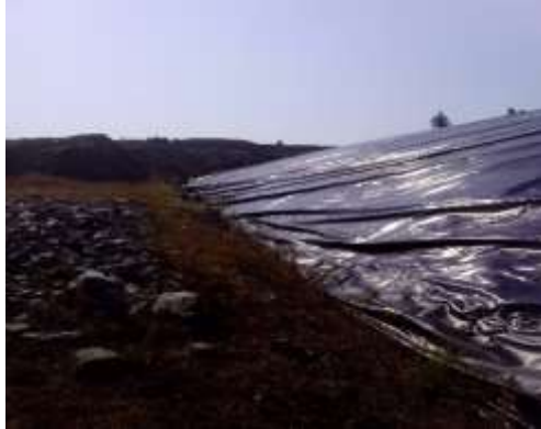
PEA – liner near NE corner
