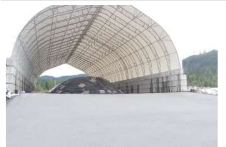
SMA - looking south
