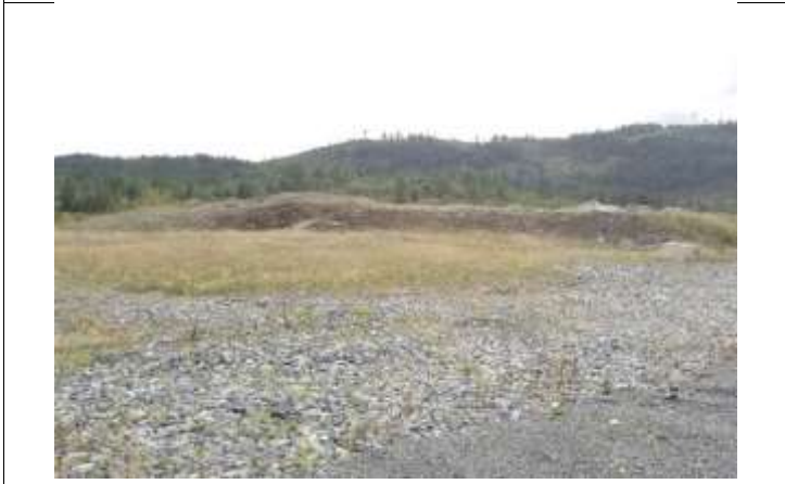
Contact water containment Pond
