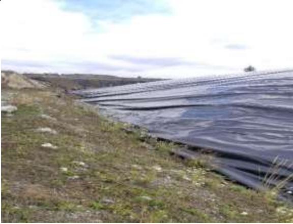
PEA – liner near NE corner
