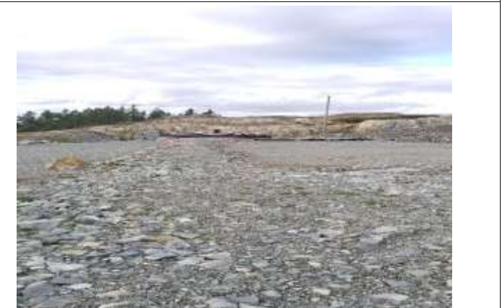
Leak and leachate detection works
