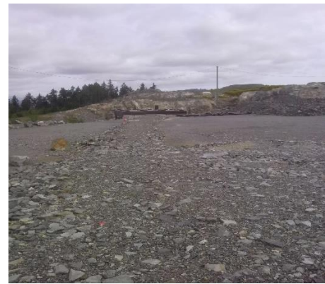
Pipe trenching and Leachate and Leak Detention facility
