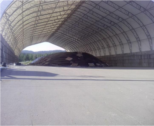
SMA - looking south
