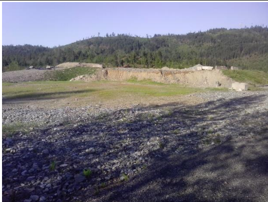
Contact water containment Pond
