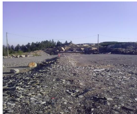
Leak and leachate detection works
