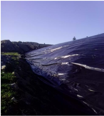
PEA – liner near NE corner
