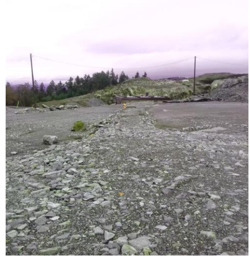
Leak and leachate detection works
