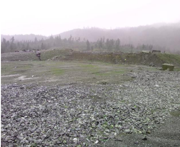
Contact water containment Pond
