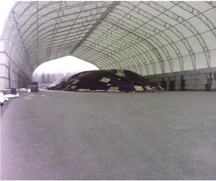
SMA - looking south
