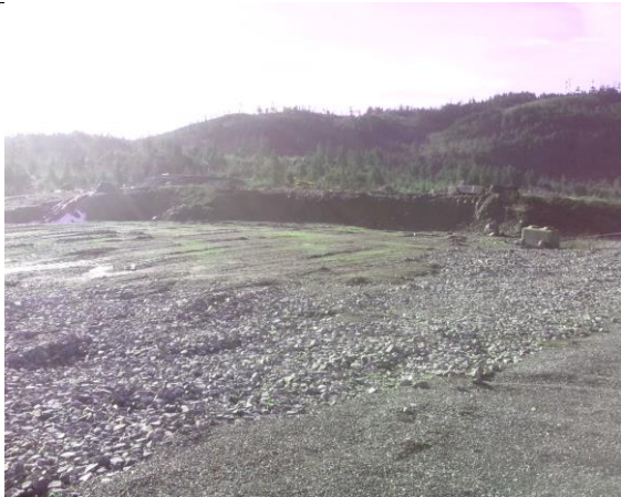
Contact water containment Pond
