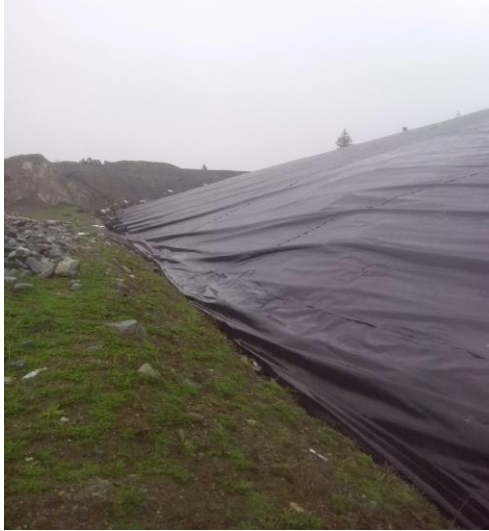
PEA – liner near NE corner
