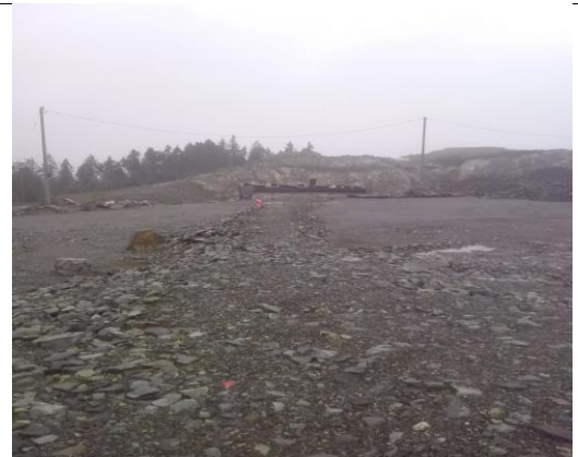
Pipe trenching and Leachate and Leak Detention facility
