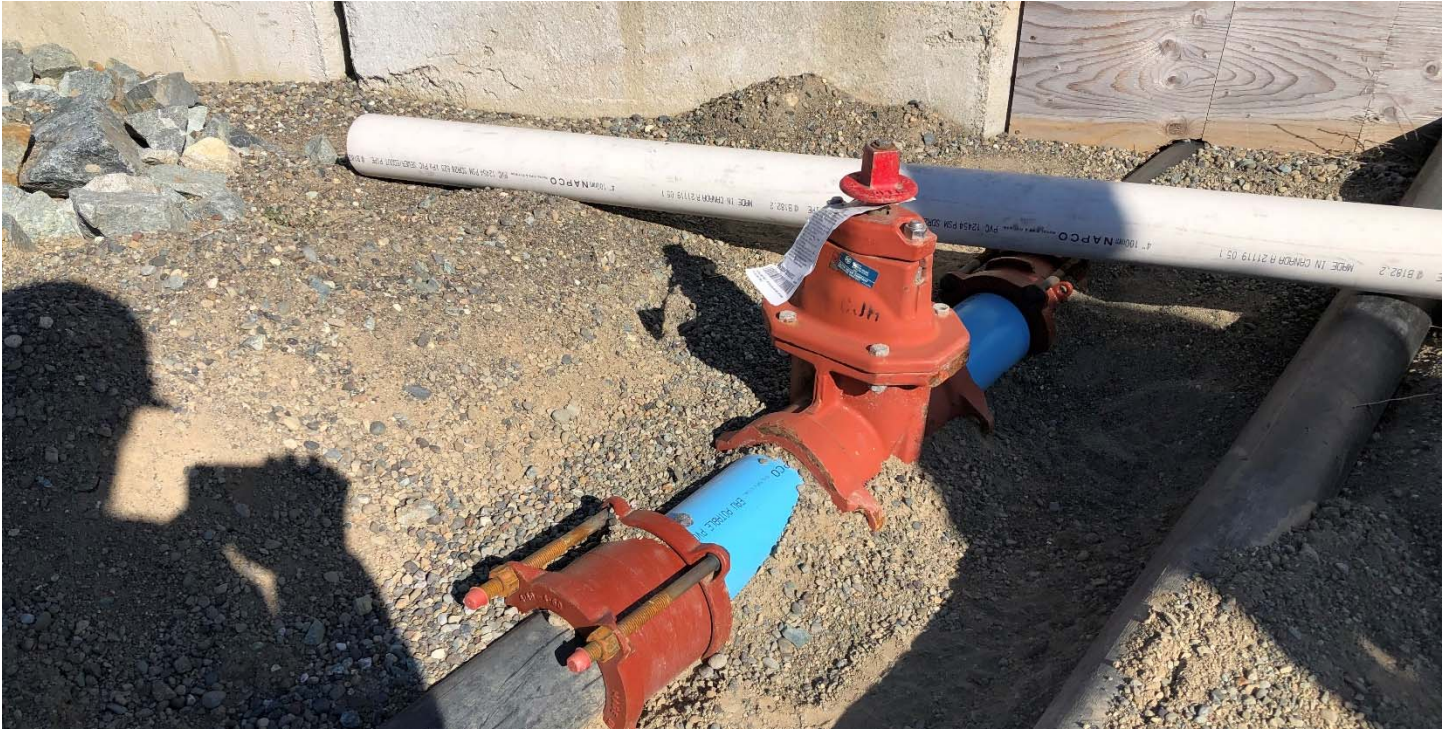
Picture #11: Allterra installed a leachate pipe valve at the south side of the Leachate Storage Facility. This valve has replaced the existing leachate pipe valve located midway between the Leachate Storage Facility and PEA.
