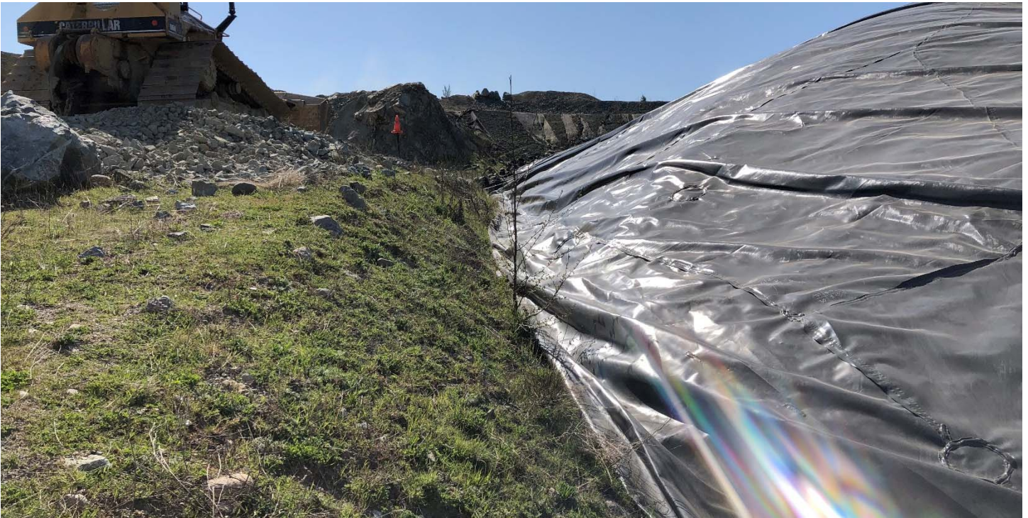
Picture #14: Soak away trench on the east side of the PEA has not been developed yet. Soakaway design for this area to be discussed.
