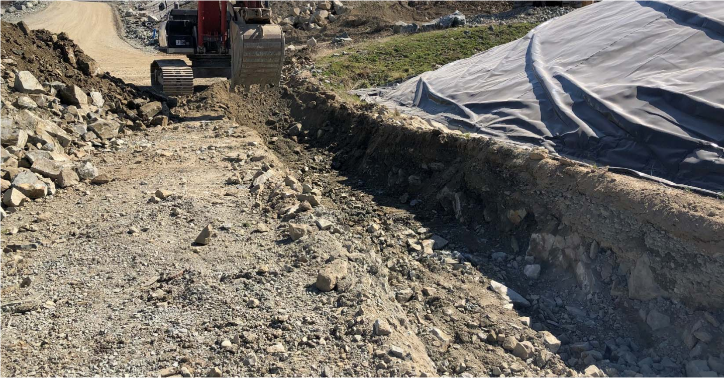
Picture #9: Allterra excavating soak away trench at north west toe of PEA.
