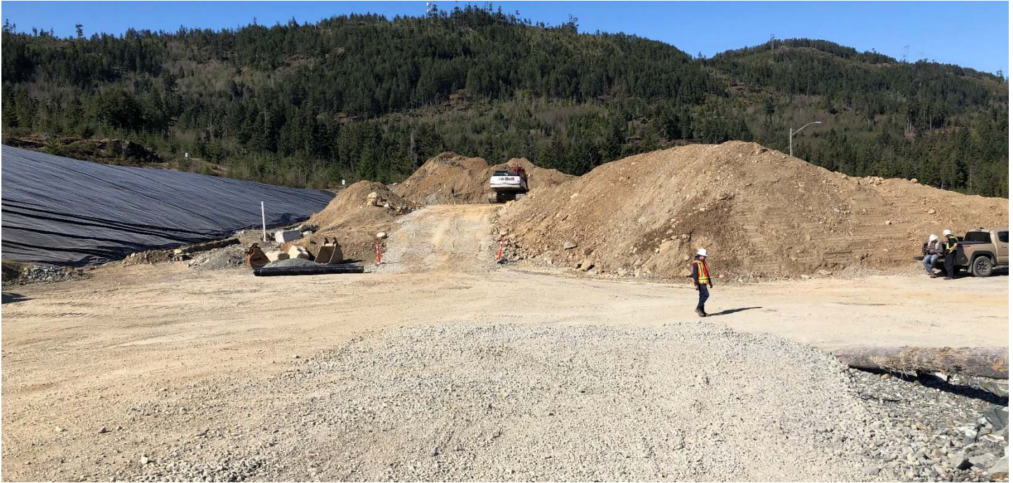
Picture# 15: Fill material stockpiled on the north side of the PEA.
