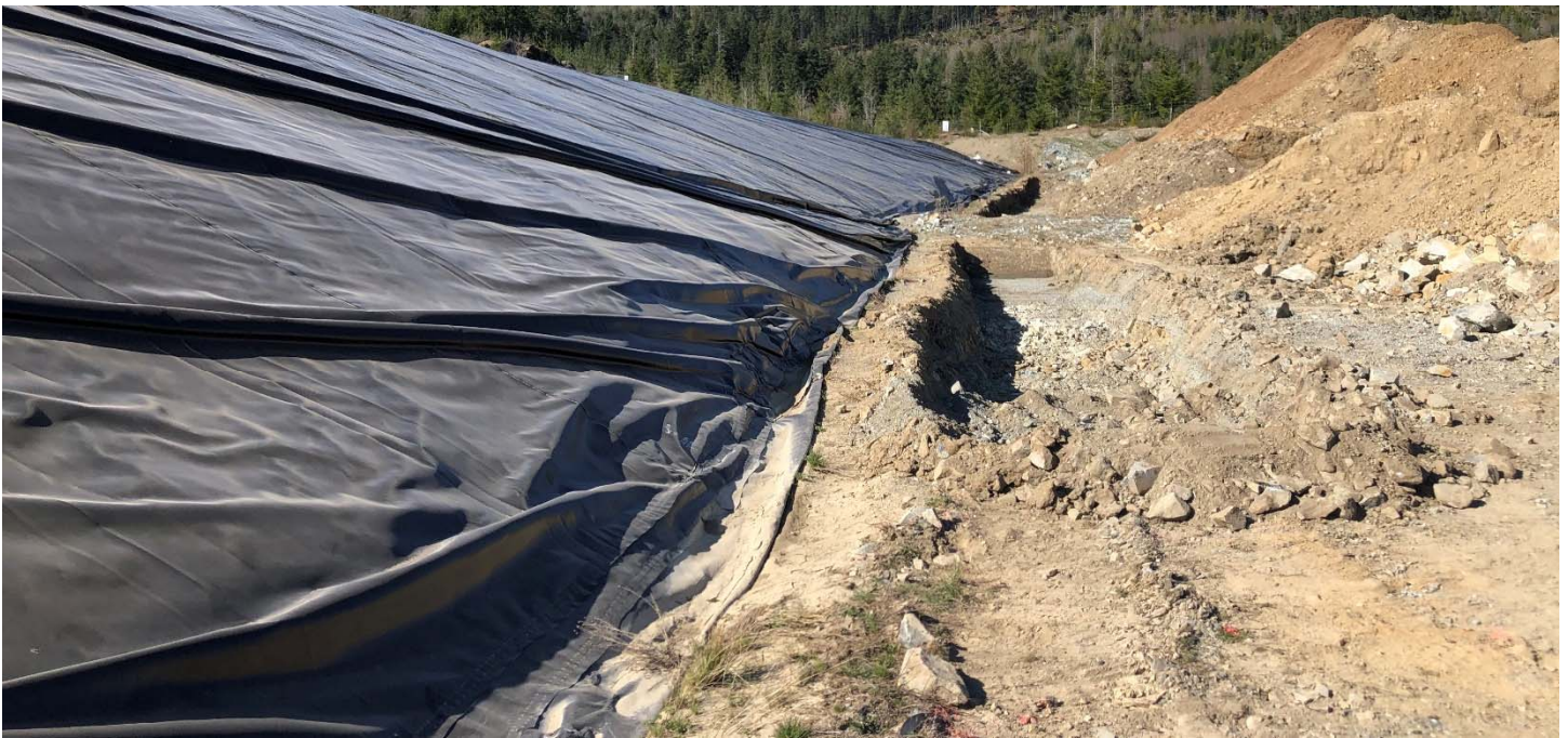
Picture #8: Soak away trench excavated along north toe of the PEA. SHA confirmed that the trench is 2 metres wide by 1 meter deep, as per design.
