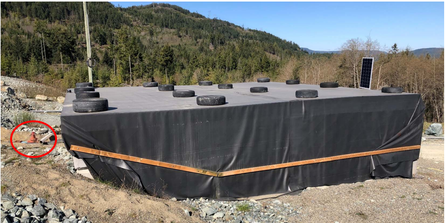
Picture #12: New valve location at south side of Leachate Storage Facility.
