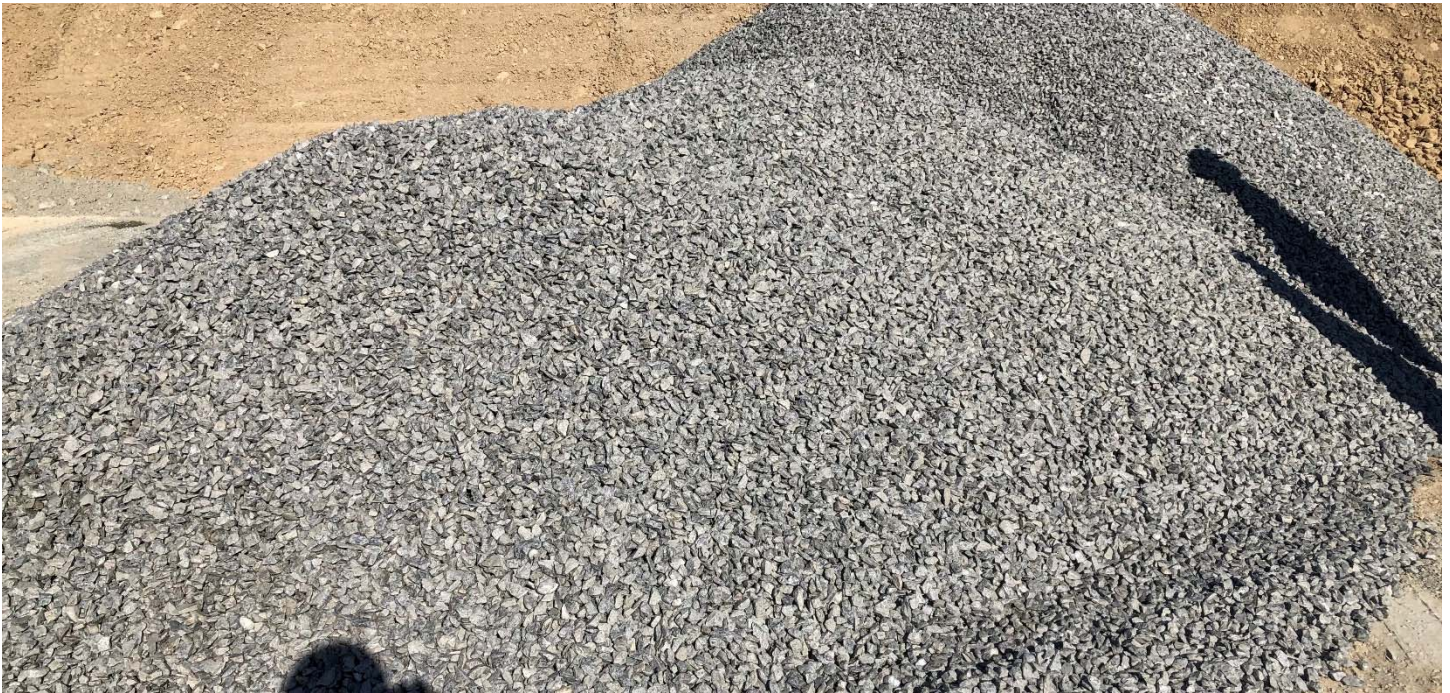
Picture # 1: SHA visually inspected the stockpile of proposed clear crush drainage gravel. SHA visual inspection of the material confirmed that the rock is uniform in quality, angular in nature, and free from excesses of flat and elongated particles, organic material, salt, and foreign objects. The material appears to be washed to eliminate fines. The material appears suitable for proposed use as the 200 mm thick drainage layer in the permanent encapsulation area (PEA) cover system.
