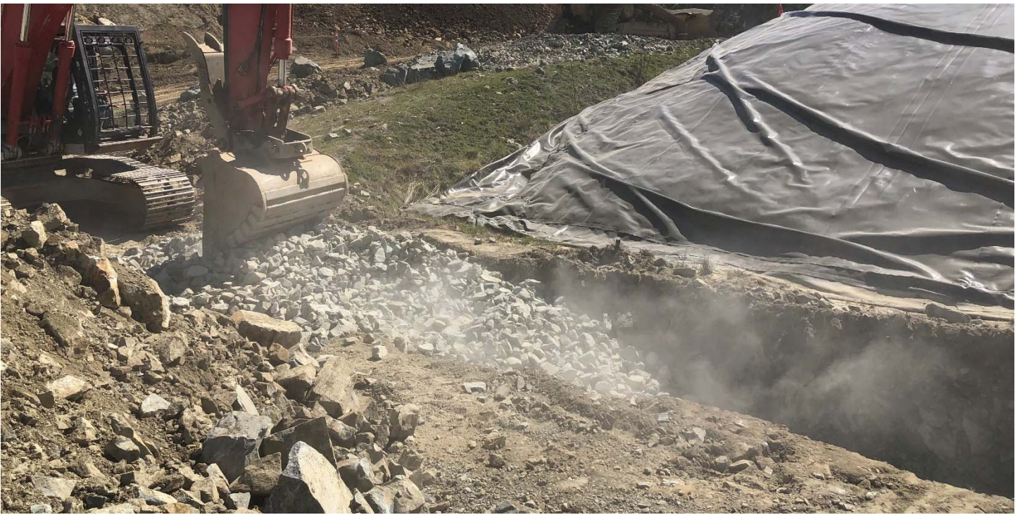
Picture #10: Allterra backfilling soakaway trench with blast rock, starting at the northwest toe of the PEA.
