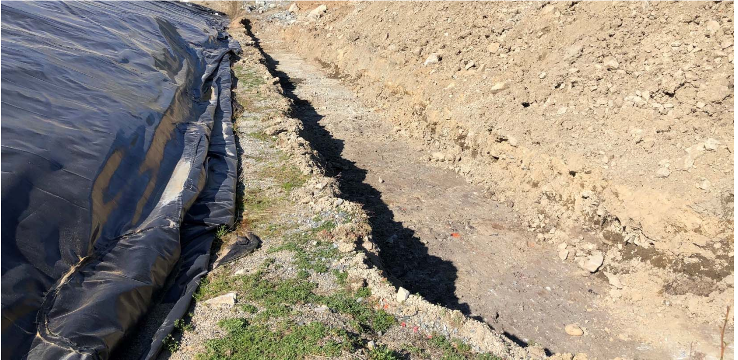
Picture #7: Soak away trench excavated along north toe of the PEA. SHA confirmed that the trench is 2 metres wide by 1 meter deep, as per design.
