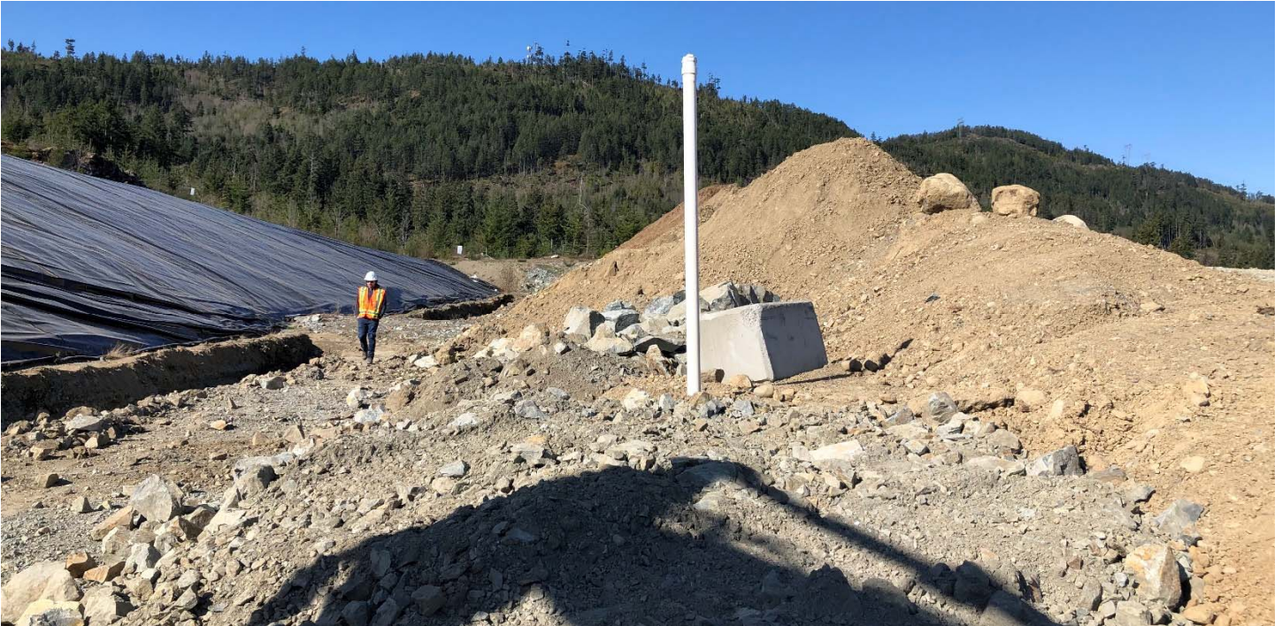
Picture #13: Allterra installed groundwater well extensions on existing groundwater wells.
