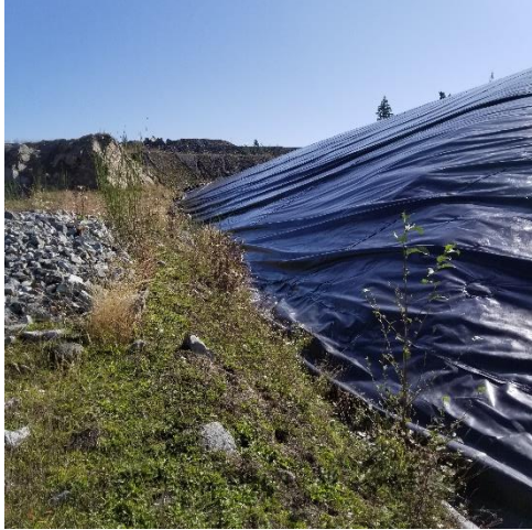
PEA – liner near NE corner
