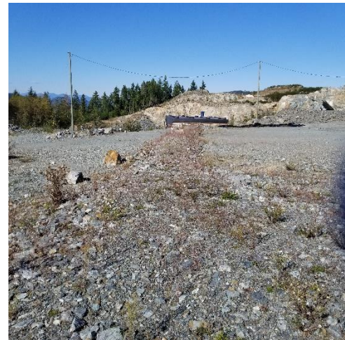
Leak and leachate detection works
