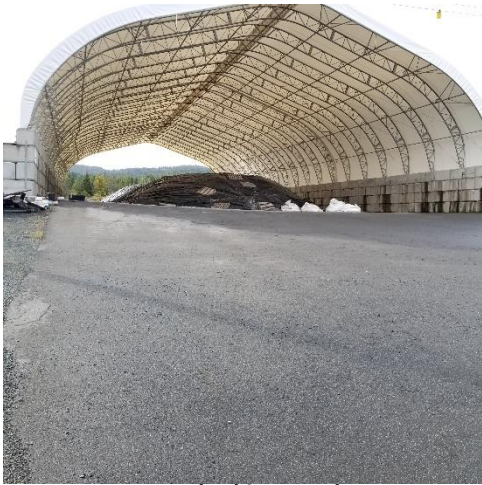
SMA - looking south
