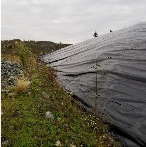
PEA – liner near NE corner
