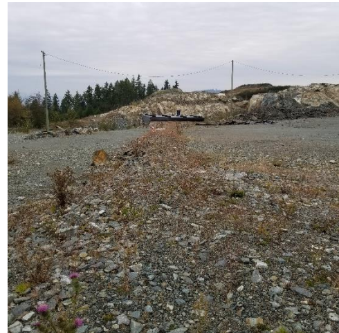
Leak and leachate detection works
