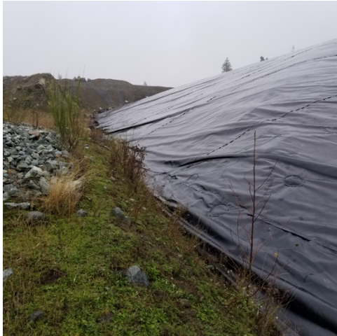
PEA – liner near NE corner
