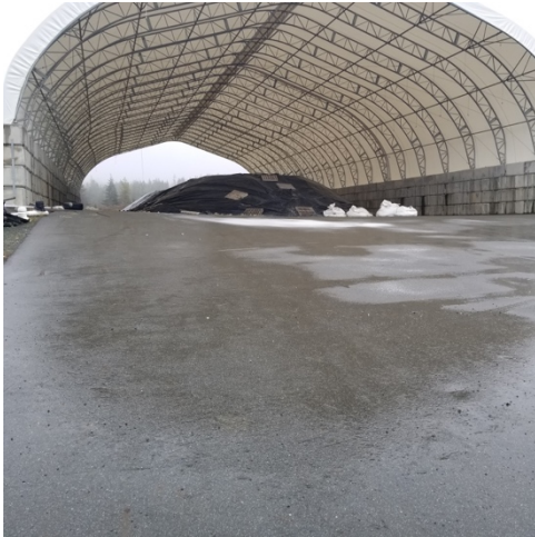
SMA - looking south
