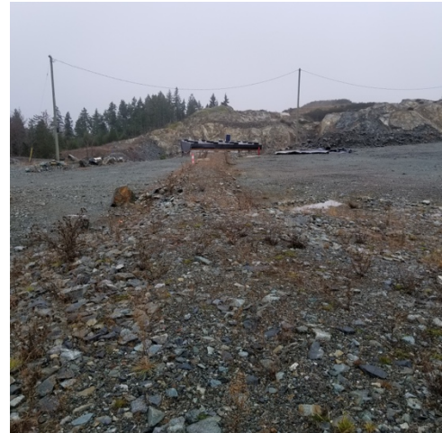
Leak and leachate detection works
