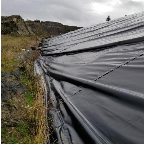
PEA – liner near NE corner
