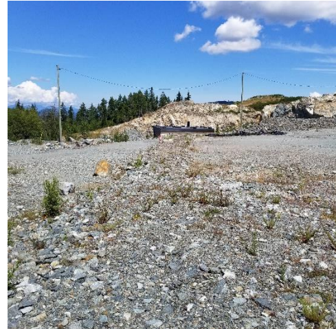
Leak and leachate detection works
