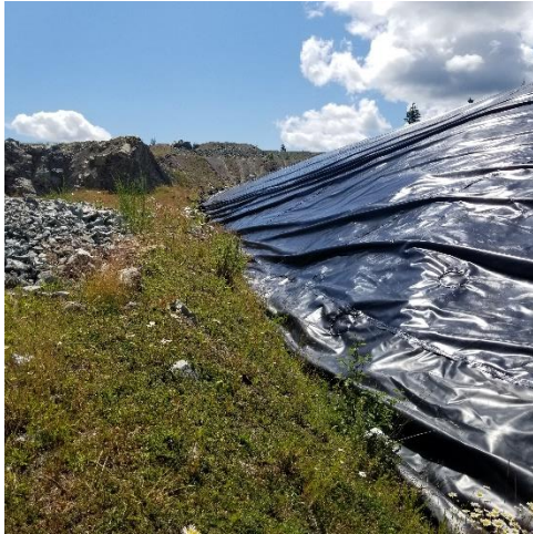
PEA – liner near NE corner
